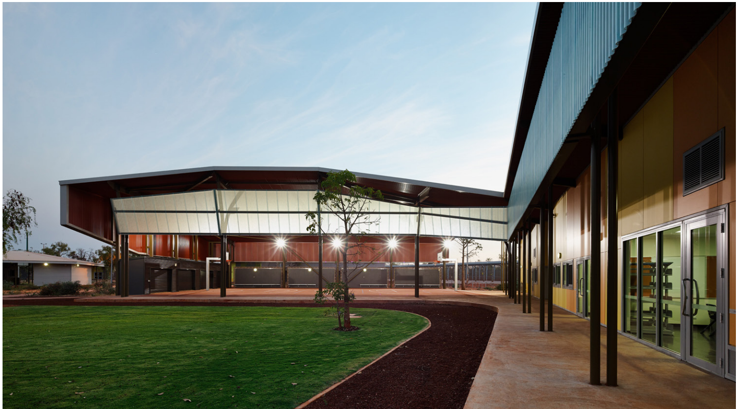
Figure 2. West Kimberley Regional Prison by TAG Architects
