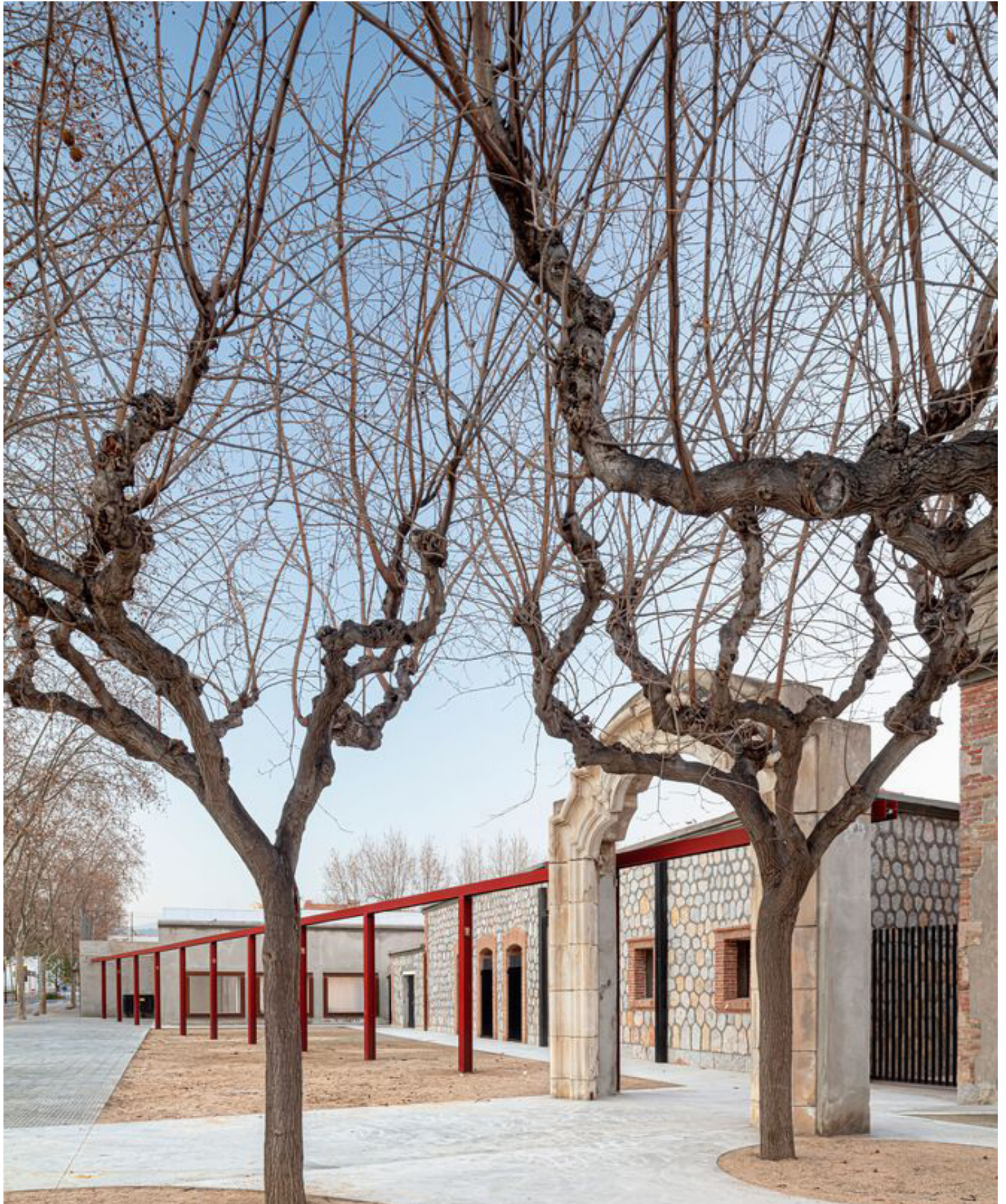
Figure 26. El Roser Social Centre - a social integration center located in an old prison building in Catalonia. Photo: Adrià Goula
